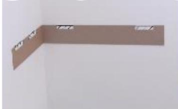
1. Using the supplied template mark the position of the grooves.
