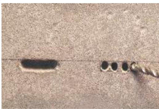
Use the small drill and drill bit. Start to drill an angle to drill out the material between the holes.
