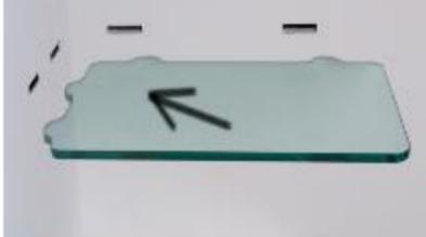
2. Use wall-saw to cut the grooves on the wall to insert the shelf.
